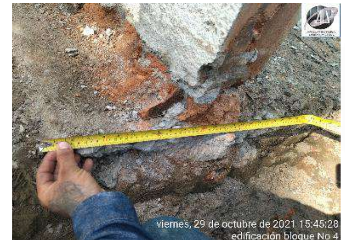
REVISION AREA DEMOLIDA
