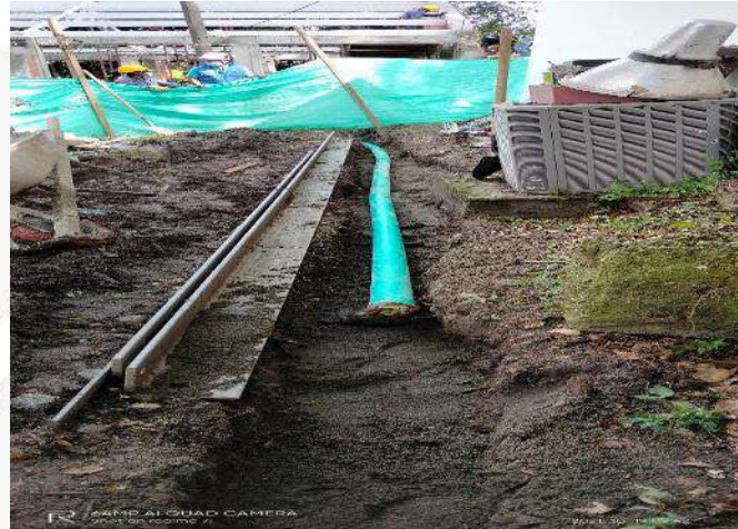
INSTALACION TUBERIA ELECTRICA EXTERNA
