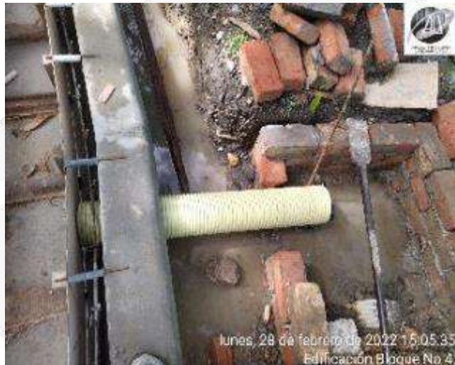
INSTALACION TUBERIA DESAGUE CARCAMO PERIMETRAL
