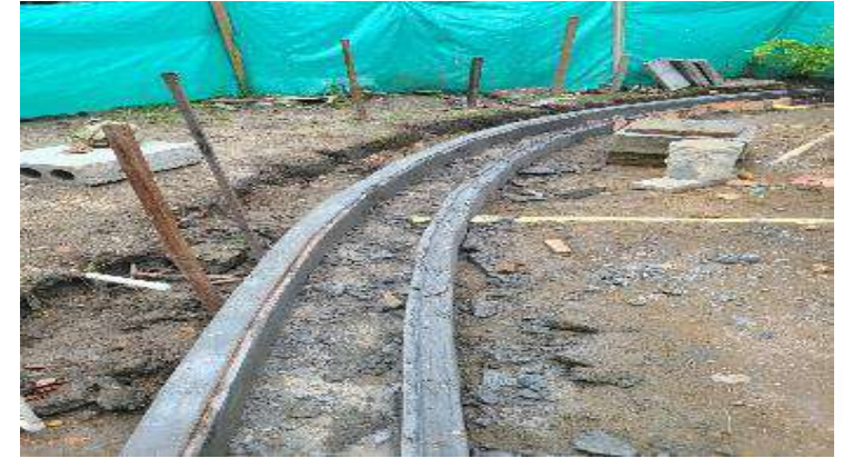
CONSTRUCCION CARCAMO PERIMETRAL
