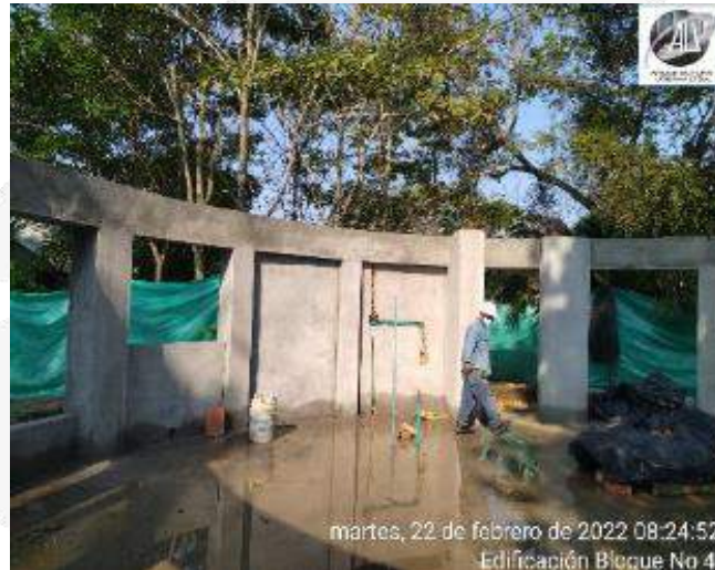
INSTALACION TUBERIA ELECTRICA
