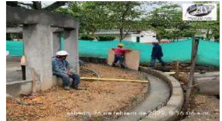
CONSTRUCCION CARCAMO PERIMETRAL
