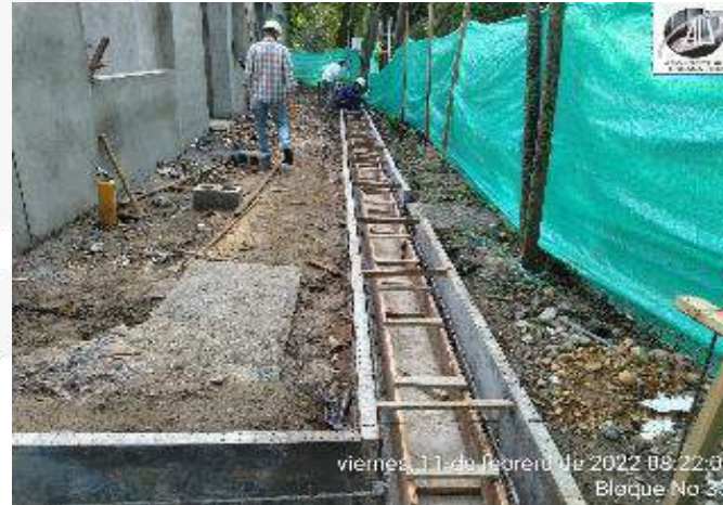
CONSTRUCCION CARCAMO PERIMETRAL
