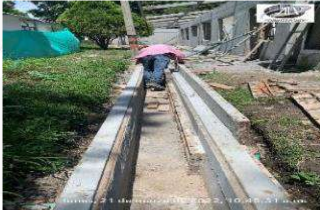
CONSTRUCCION CARCAMO PERIMETRAL
