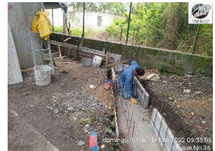
CONSTRUCCION CARCAMO PERIMETRAL
