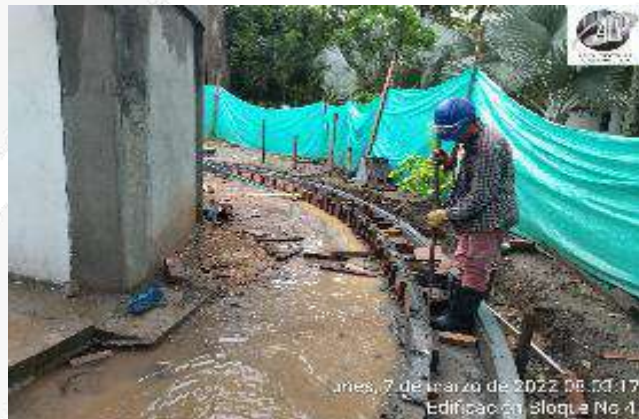
CONSTRUCCION CARCAMO PERIMETRAL
