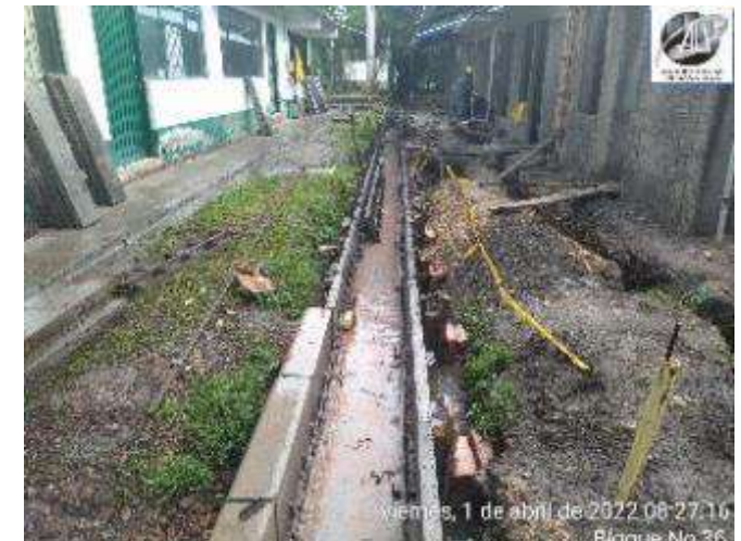
CONSTRUCCION CARCAMO PERIMETRAL
