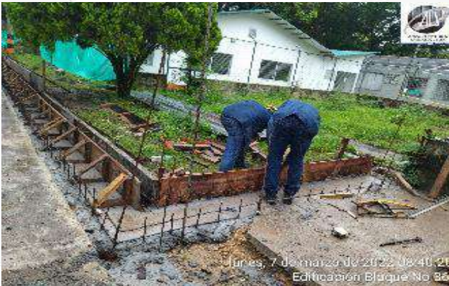
CONSTRUCCION CARCAMO PERIMETRAL
