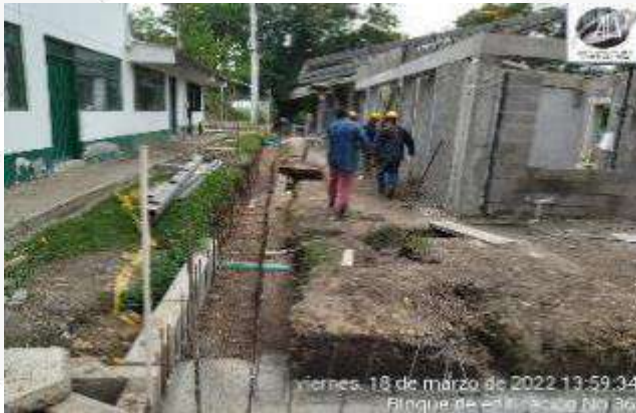
CONSTRUCCION CARCAMO PERIMETRAL
