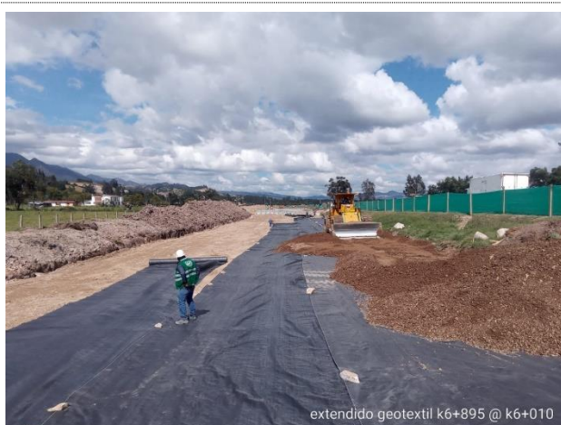
extendido geotextil k6+895 @ k6+010
