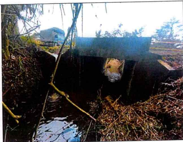
Vista trasera boxculvert
