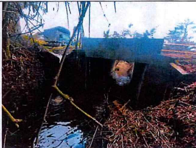
Vista trasera boxculvert
