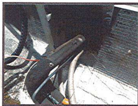
INSTALACION DE BYPASS
