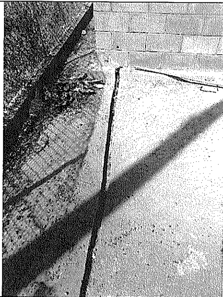
TUBERIA EMT 1/2, ACOM.E 3F(3#4/0+1#4/0)3", SAL LAMP EMT
