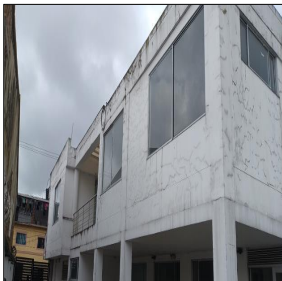
Fachada Principal Interna
