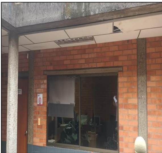
Cielo Raso Corredor Patio Central
