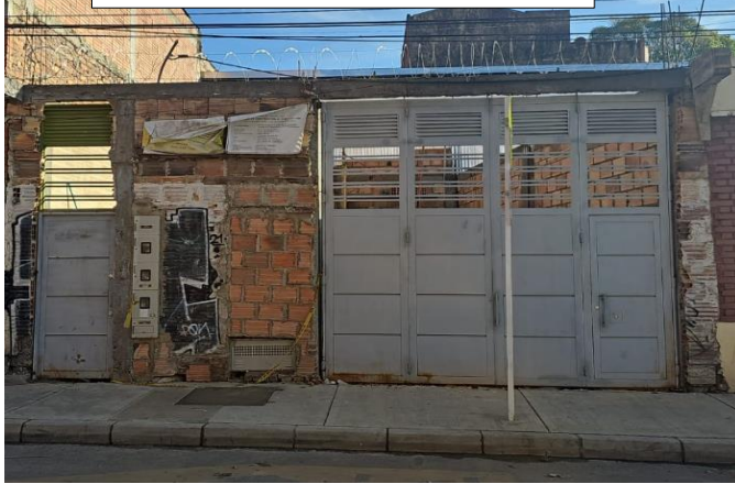
FOTO FACHADA PRINCIPAL 17-10-2024
