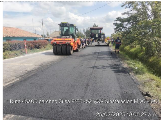
PR28+0521 – PR28+0545, Susa, fresado e instalación de MDC-19 (25/02/25)
