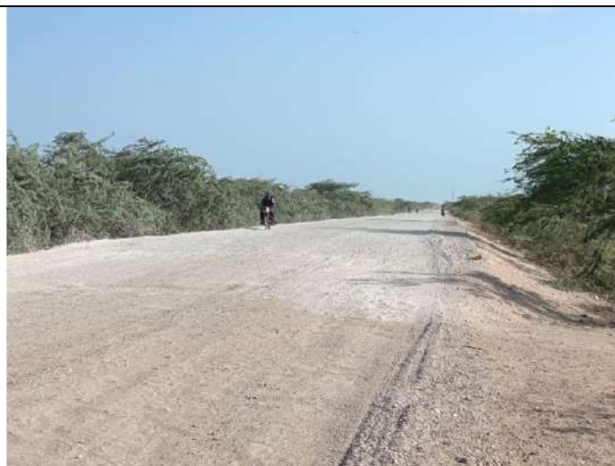
Subbase granular Pr +101+220
