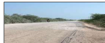
Subbase granular Pr +101+220
