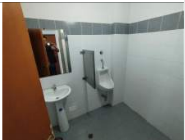
VISTA GENERAL BAÑOS
