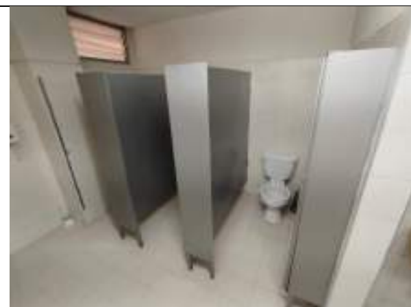
VISTA GENERAL BAÑOS
