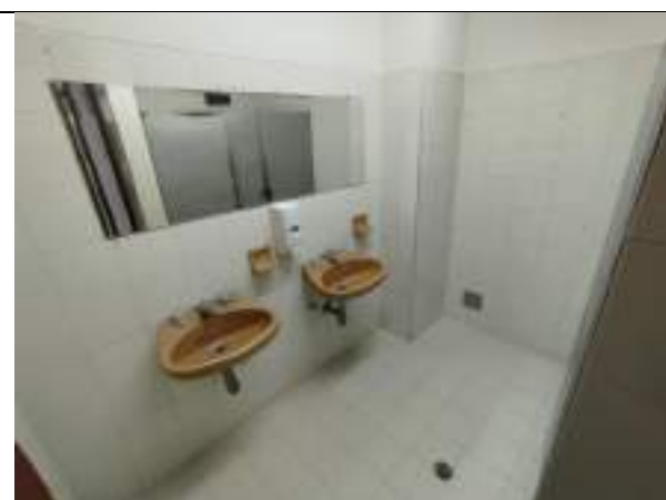
VISTA GENERAL BAÑOS
