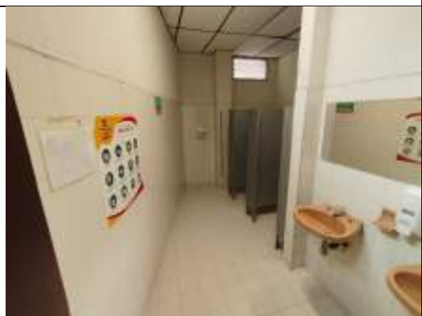
VISTA GENERAL BAÑOS
