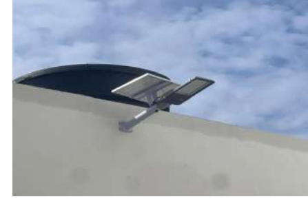
INSTALACION DE LUMINARIA SOLAR LED LIGHT SOLAR S50 KIT
