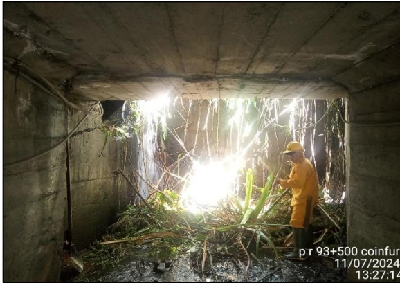
PR93+0500. Limpieza de box coulverts.
