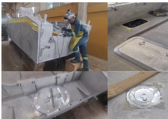
Foto No. 49 a 52 – Bote No. 5, 6, 7 y 8 Outfitting, manholes y handholds
