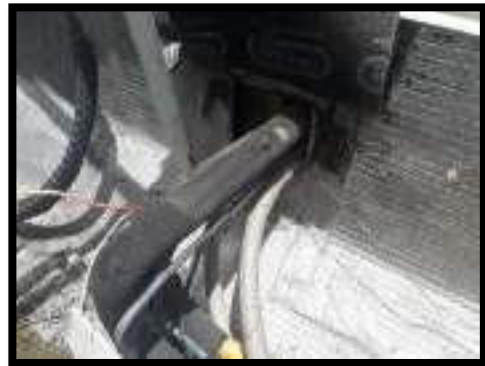
INSTALACION DE BYPASS
