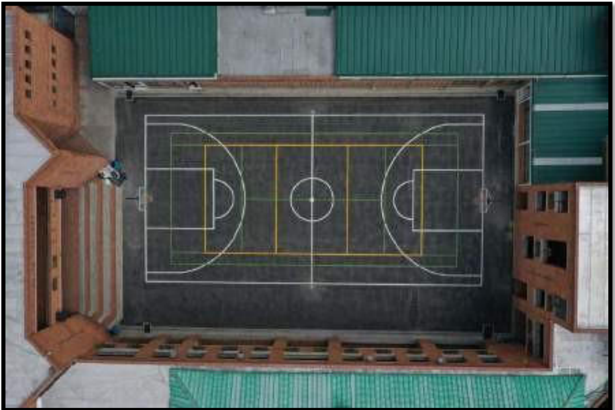
ACABADO FINAL CANCHA MULTIPLE
