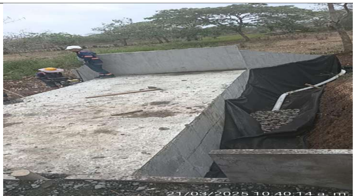
Box Culvert PR35+430. Filtro lateral sentido sur-muro 1.
