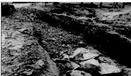
RELLENO DE CAJA PR2+215, PR2+240 BOXCULVERT
