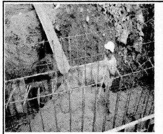
FUNDIDA PISO BOX COULVERT PR 4+820
