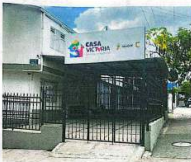
Entrada Principal Casa victoria
