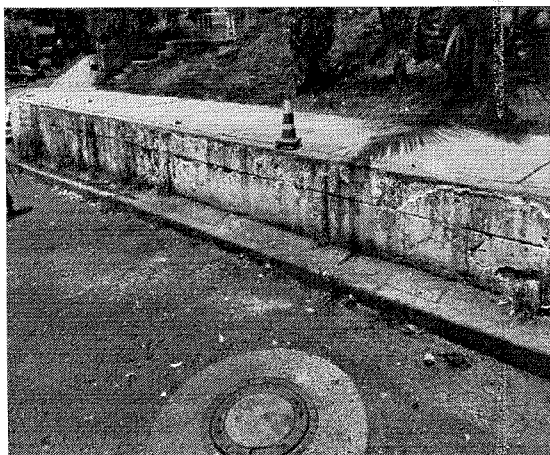
Entrega Pluvial a BoxCulvert – 2.25m * 3.30m
