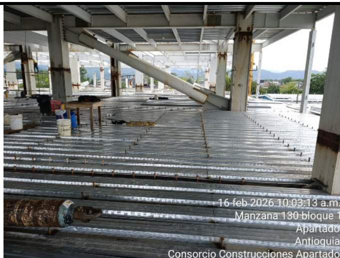
Instalacion steel deck Torre Medica
