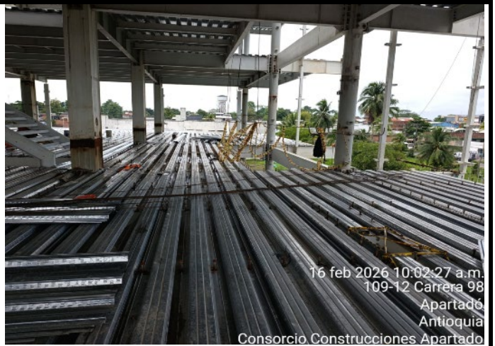
Instalacion steel deck Torre Medica
