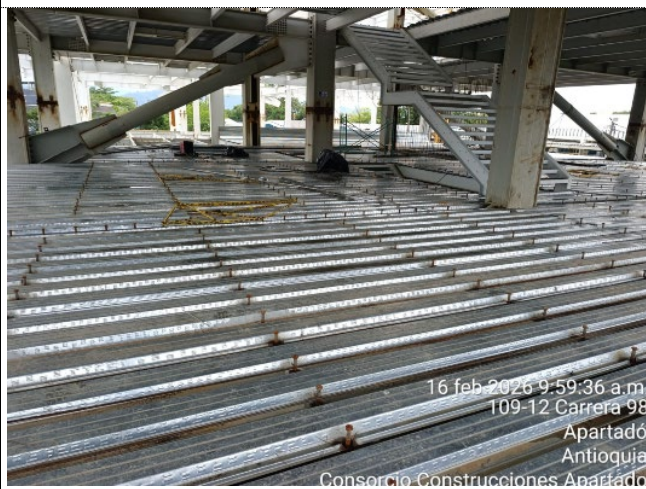
Instalacion steel deck Torre Medica
