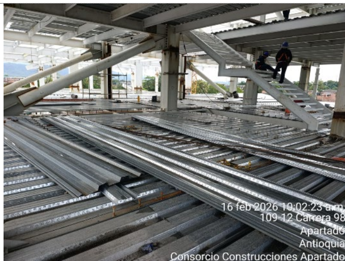
Instalacion steel deck Torre Medica
