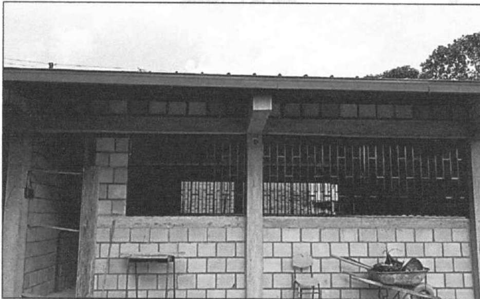
FACHADA PRINCIPAL AULA
