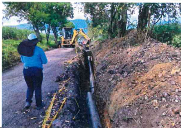
EMPALME TUBERIA PEAD 14" TRAMO 3
