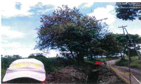
EMPALME TUBERIA PEAD 14" TRAMO 3
