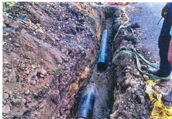
EMPALME TUBERIA PEAD 14" TRAMO 3
