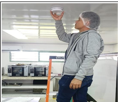
INSTALACION SENSOR CHOCOLATERIA
