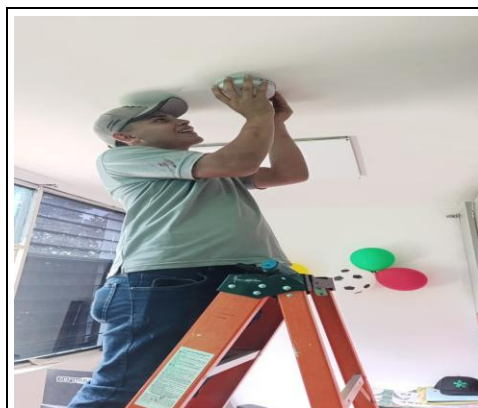
INSTALACION COORD. ACADEMICA
