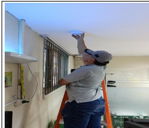
INSTALACION COORD. ACADEMICA
