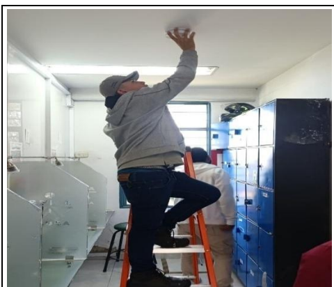
INSTALACION SENSOR CHOCOLATERIA
