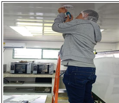
INSTALACION SENSOR CHOCOLATERIA
