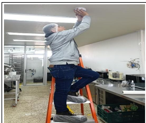
INSTALACION SENSOR CHOCOLATERIA
