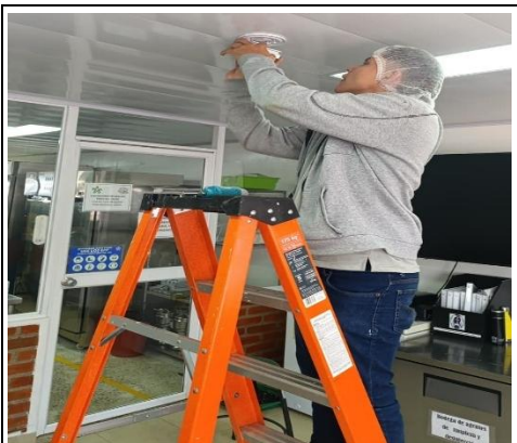
INSTALACION SENSOR CHOCOLATERIA
