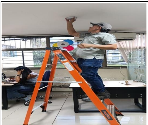
INSTALACION COORD. ACADEMICA
