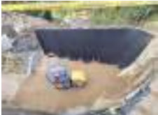
RELLENO SUBBASE GRANULAR
