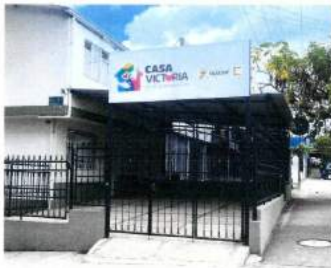
Entrada Principal Casa victoria
