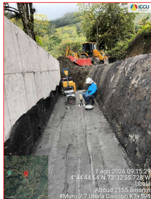
Relleno estructural k7+424
