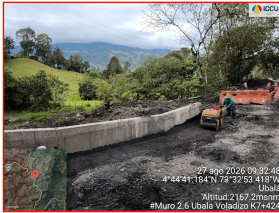
Relleno estructural k7+424
