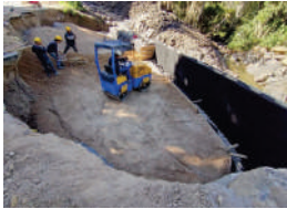
RELLENO SUBBASE GRANULAR
