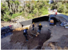
RELLENO SUBBASE GRANULAR
