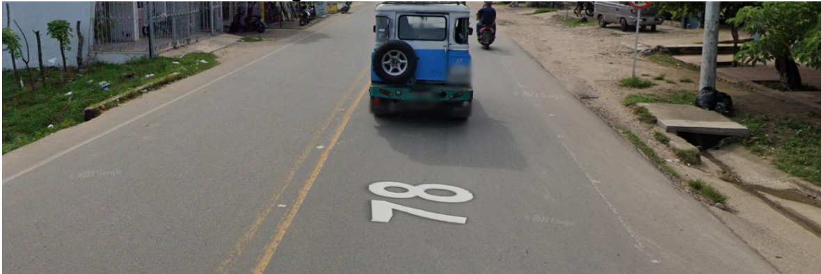
Figura 6. Box culvert K0+145
